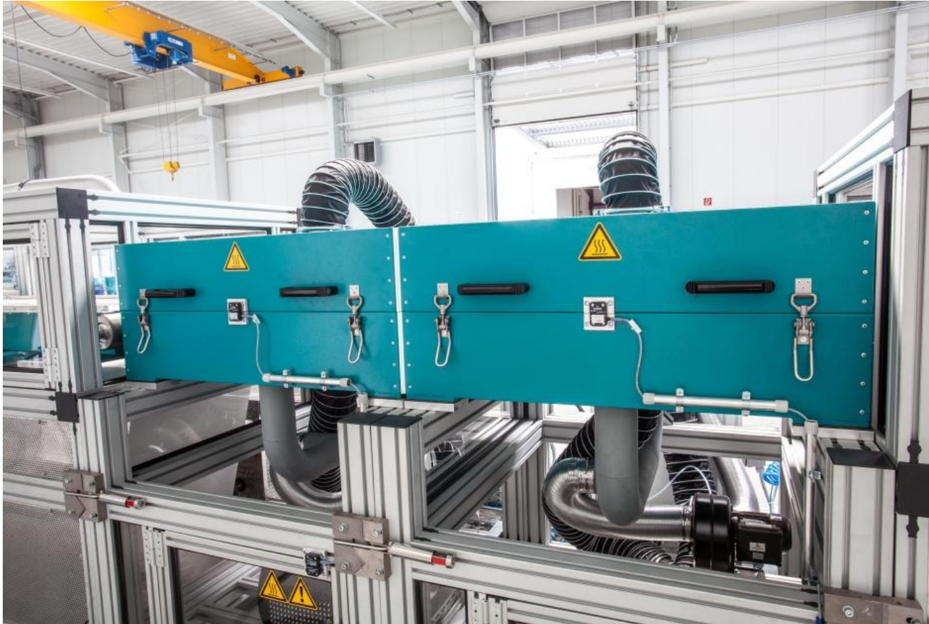
7. Dryer with fan air supply heater
